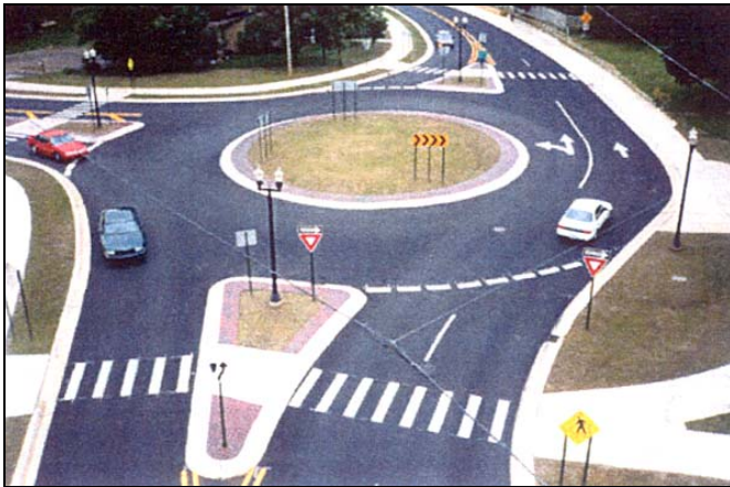
Figure 8.8 Modern, low-speed roundabout (DLZ Engineers)
