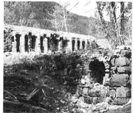
View of coke ovens
