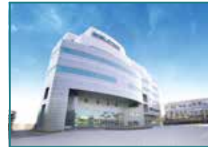
Mobiletron (Taiwan) • Taichung
