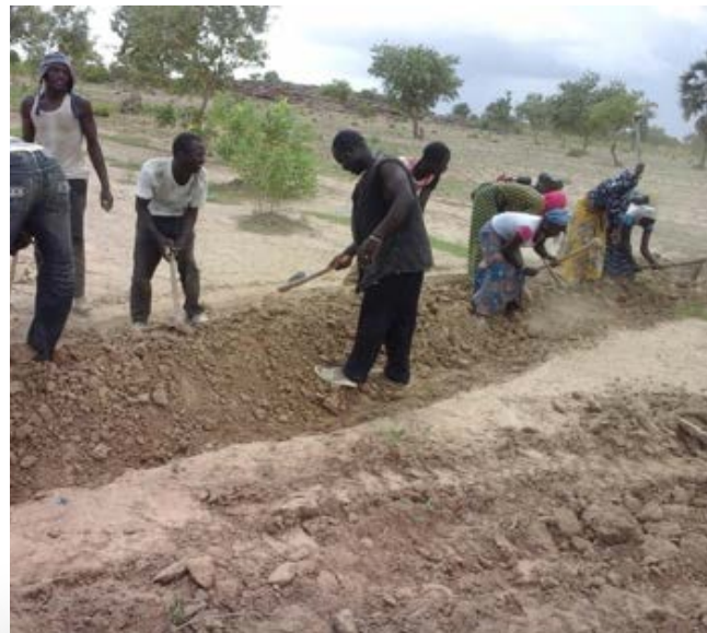
Figure 4.2: Earth-bunds technique for water collection around trees and for the rehabilitation of degraded lands in Koe-Doe Mopti, Mali (Source: Ouodiouma Samake, World Agroforestry).
