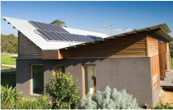
← Cover image by Lindsay Edwards Photography. Tim Adams designed the roof of his house to maximise the effectiveness of solar PV. Page 34
