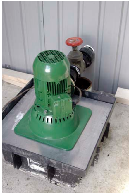
↑ The Platypus Power micro-hydro turbine provides a large proportion of the lodge's electricity.
