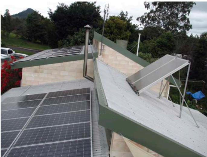
↑ The roof features two solar PV arrays, solar water heating system, the flue for the AGA stove and a white vent for the composting toilet.
