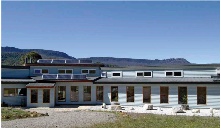
↑ Forest Walks Lodge sources its electricity from a combined solar and micro-hydro system.
