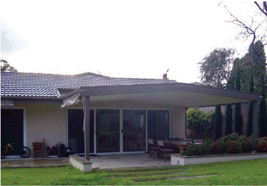
↑ The roofed outdoor area provides protection for the family room from the elements and the sun. Drop-down blinds on the western side provide additional shading during summer.
