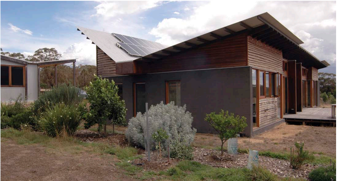
↑ The roofline of the house was designed specifically to provide the optimum angle for the north-facing solar panels.
