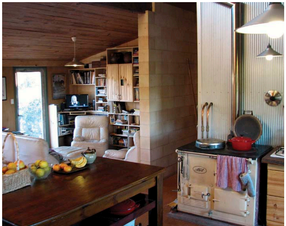
↑ Features in the kitchen and living area include an AGA combustion stove, LED lights, an energy-efficient TV and an internal block wall for thermal mass. The inverter is mounted behind the doors in the bookcase.
