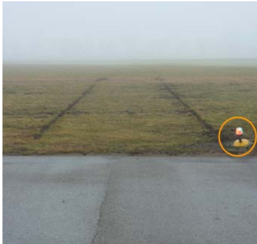
Figure 1: View in the direction of departure at the end of runway 07. In the foreground on the right: the end-of-runway light which was struck (circled in orange).
