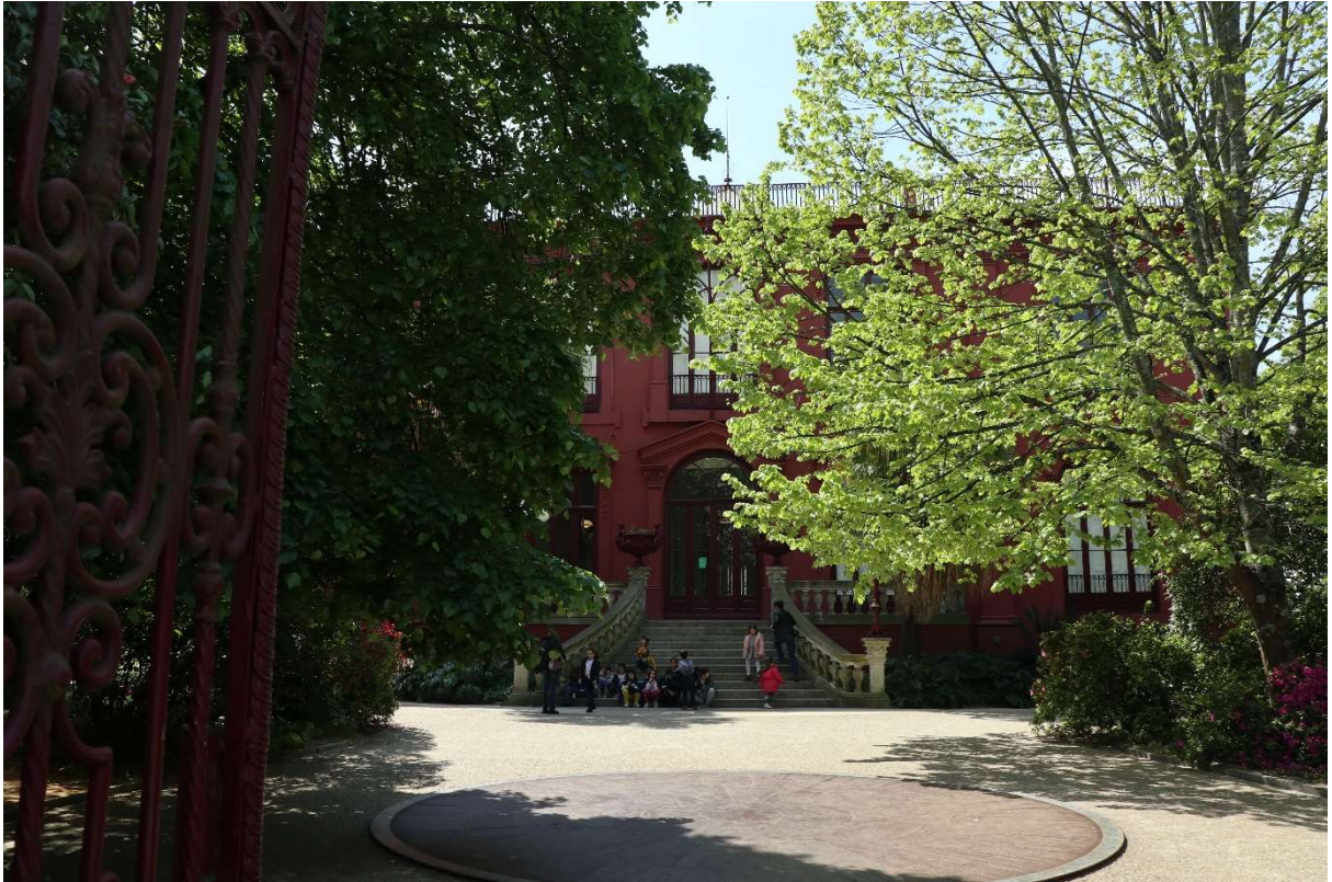
Main entrance of Hall of Biodiversity.
