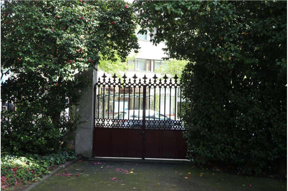
Entrance at the intersection of the Rua do Campo Alegre with Travessa de Entrecampos.
