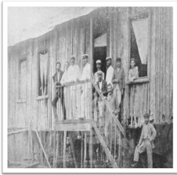
Figure 36. Offices of the National Delegation in Puerto Acre c. 1900
