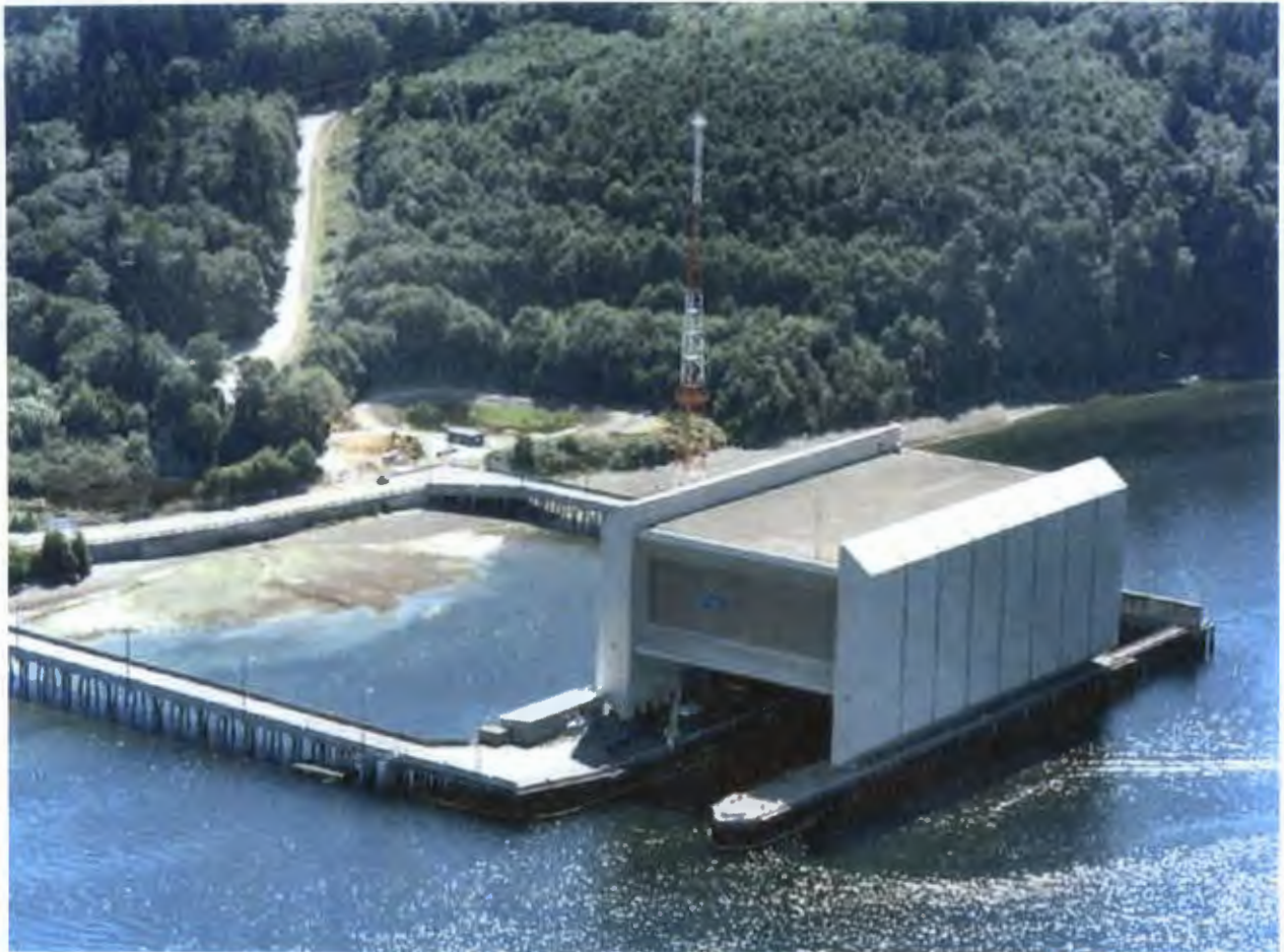
Explosive Handling Wharf-1
