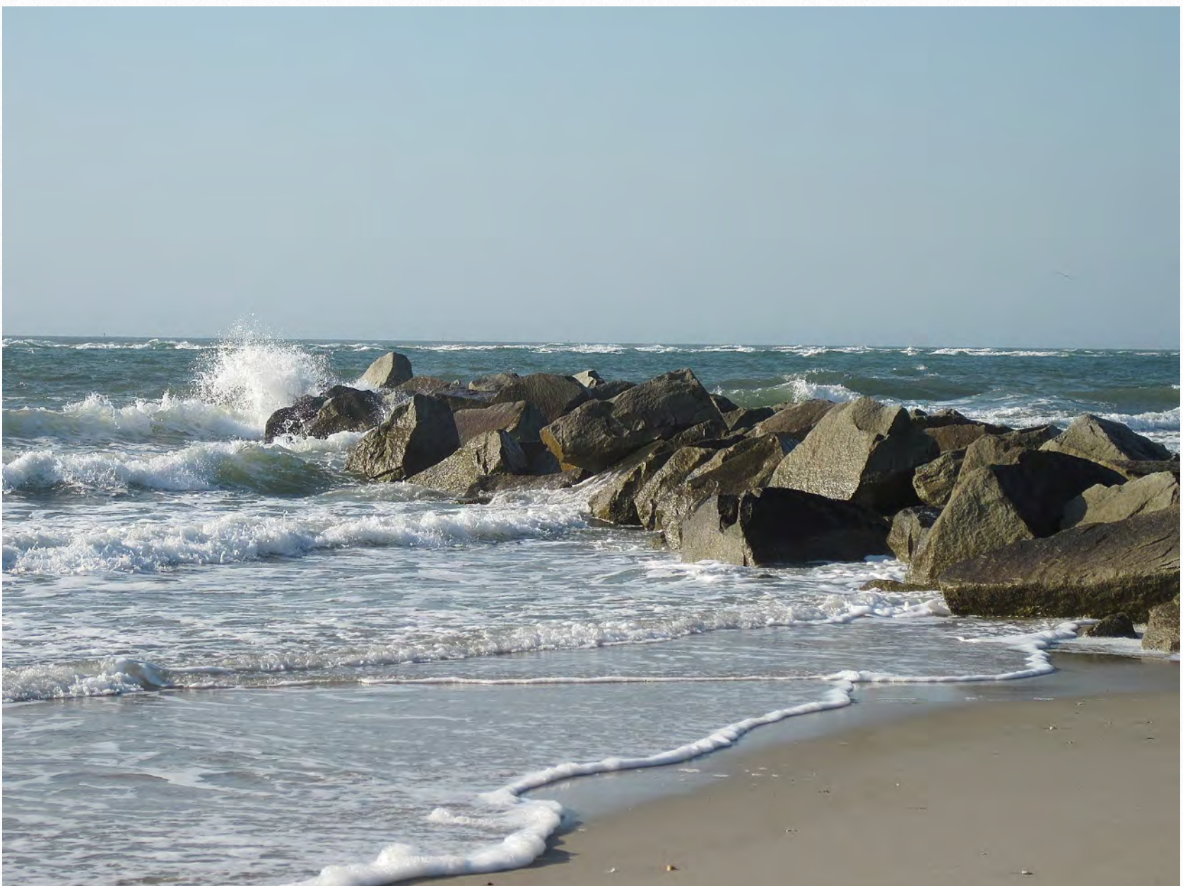
Jetty at Fort Macon, NC Image by Humberto Diaz
