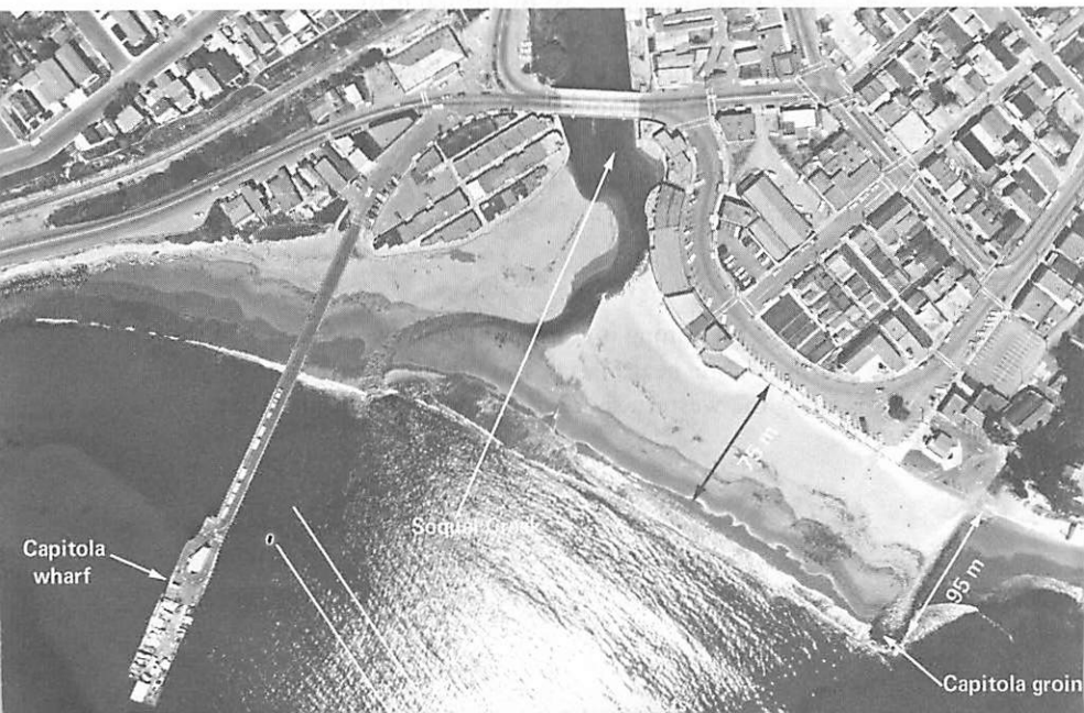
Capitola groin in April, 1971 (completed in July, 1970). Capitola beach is replenished by littoral drift trapped on the upcoast side of the groin. (Photo, U.S. Army Corps of Engineers)
