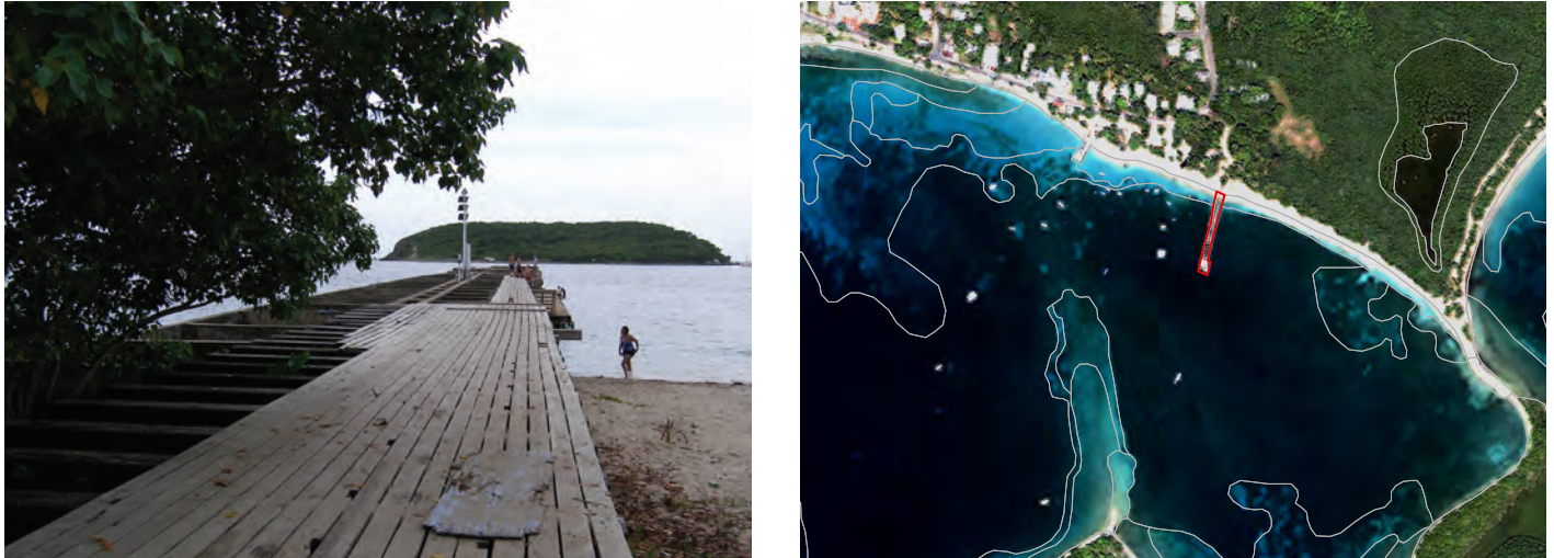
Figure 2.23. Depictions of the pier in Esperanza, an Artificial structure in Vieques. A red polygon outlines the feature on satellite imagery.
