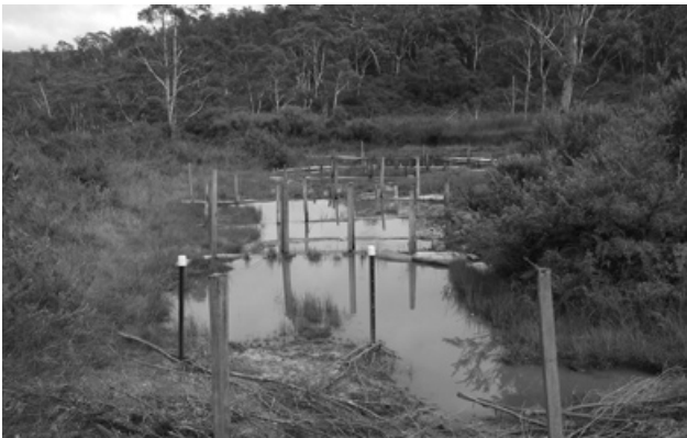
Infiltration cells rehydrate swamp areas degraded by recreational vehicle damage, Newnes Plateau. Photo: Michael Hensen.
