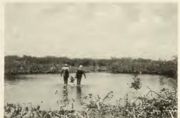
**Figure 3.** Crossing Hummingbird Pond (between cores 13 and 14 on Figure 1) with vibracore unit. The tripod can be seen at site 14 in the background.
