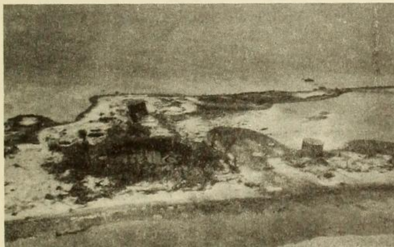
c. Aerial view of Sydneytown area showing large tank surrounded by rubble embankment covered by vegetation and two smaller tanks which have been moved by the storm waves from the two circular foundations visible just beyond the farther tank. Scour channel across reef to left of nearer small tank. (Gressitt photo).
