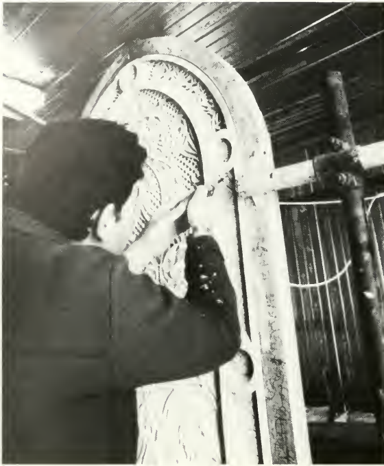
It takes Bashir more than a month to complete a window. He carves designs manually using hand tools and occasionally an electric drill, carefully slanting the angle to allow light to pass through. Photo by Joan Wolbier
