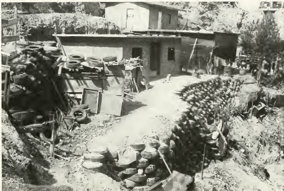
Most Mixtecos in Tijuana live in the neighborhood known as the Colonia Obrera, where retaining walls made of tires are used to keep homes from sliding down steep hills. Photo by Laura Velasco Ortiz
