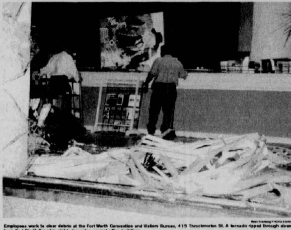
Employees work in clear debris at the Fort Worth Convention and Visitors Bureau, 415 Throckmorton St. A tornado ripped through downtown Fort Worth Tuesday night, damaging several office buildings.
