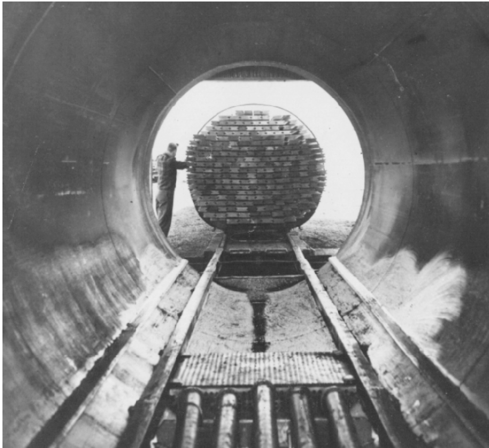
Figure 5-1. Interior view of a treating cylinder at a wood-preserving plant [121].
