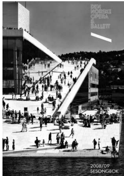
FIG. 13: Oslo Opera House after the inauguration.
