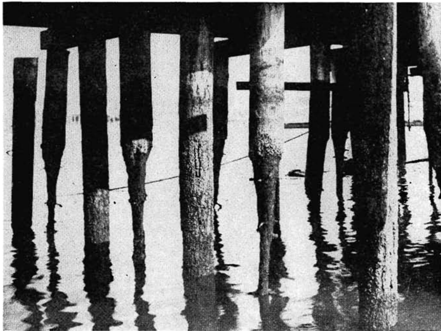
FIGURE 2. Untreated Douglas fir piling in San Francisco Bay showing the pencil-point erosion of the piling, characteristic of Limnoria attack within the intertidal zone. Photo reproduced from Hill and Kofoid, 1927, fig. 13, with permission of the University of California Press.
