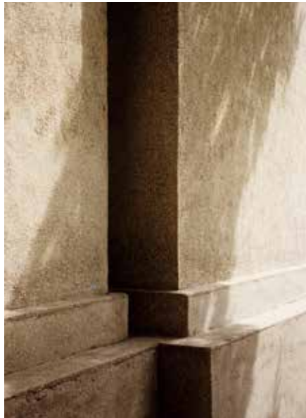
FIG. 1.5 Unity Temple. Play of contraction and expansion (ressault) at the place of the slot. [Photo: Frans Sturkenboom]
