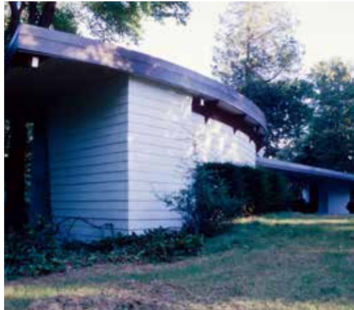
FIG. 1.50 The convex side of the Curtis Meyer House. [Photo: Frans Sturkenboom]
