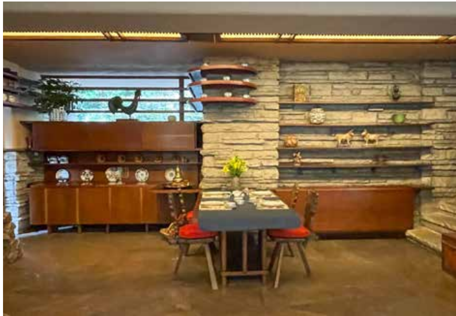
FIG. 3.31 Fallingwater. Shelves crossing different material surfaces. [Photo: Anny C. Wynn]
