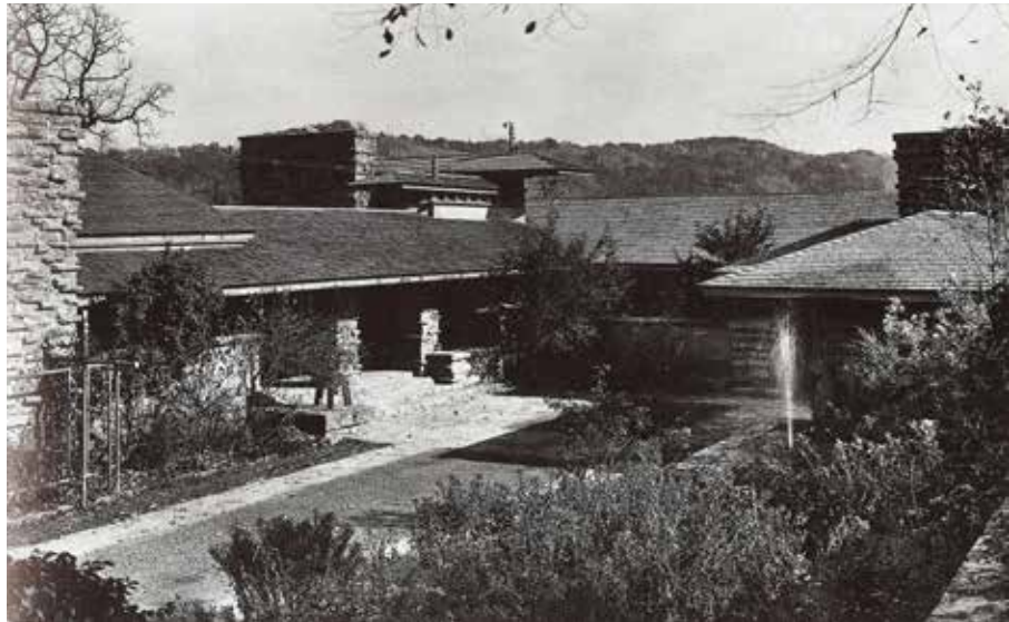
FIG. 3.15 Pagoda-like small roofs piled up on top of the architect's quarters in Taliesin II. [Courtesy of FLLWFA (MOMA / AA&FALCU)]
