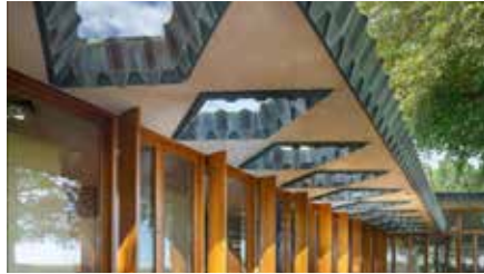
FIG. 2.34 Randall Fawcett House, Los Banos (CA), 1961: perforated eave with cornice. [Photo: Jim Gimmons, courtesy Crosby Doe Associates]
