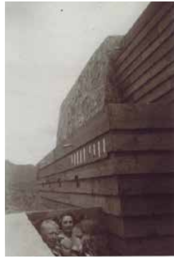
FIG. 4.35 Pauson House: overlapping board technique. [Photo: unknown]
