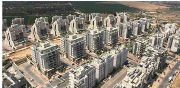
FIG. 5.64 Tzur Yitzhak as a collection of isolated buildings, 2014. (Shikun U'Binui)
