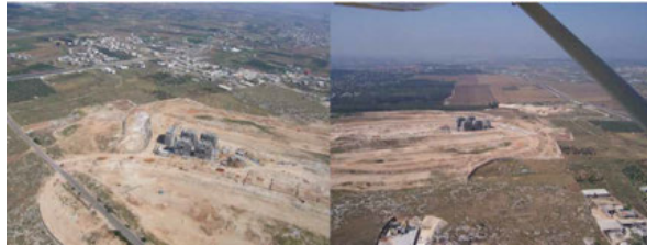
FIG. 5.53 First Project in Tzur Yitzhak, developed by the private settlers' associations, 2008 (Tzur Yitzhak Council)
