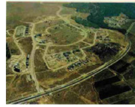
FIG. 5.36 Construction of Phase 1, 1997. (Ela'ad Council)
