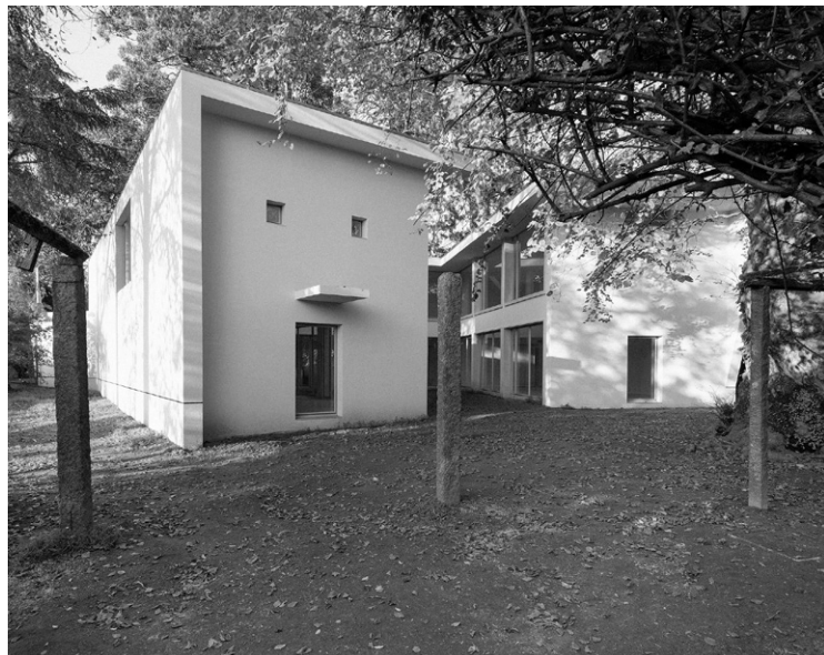
Fig. 7: Exterior view of the Carlos Ramos Pavilion
