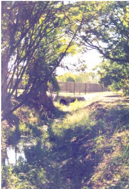
Figure 6.4 Cranbrook Creek, Cranbrook, Townsville. The creek has been modified to form a stormwater drain (note: outlet pipes in mid-background), an example of a High Disturbance habitat
