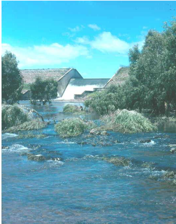
Figure 2.3 Ross River Dam spillway during the Wet Season
