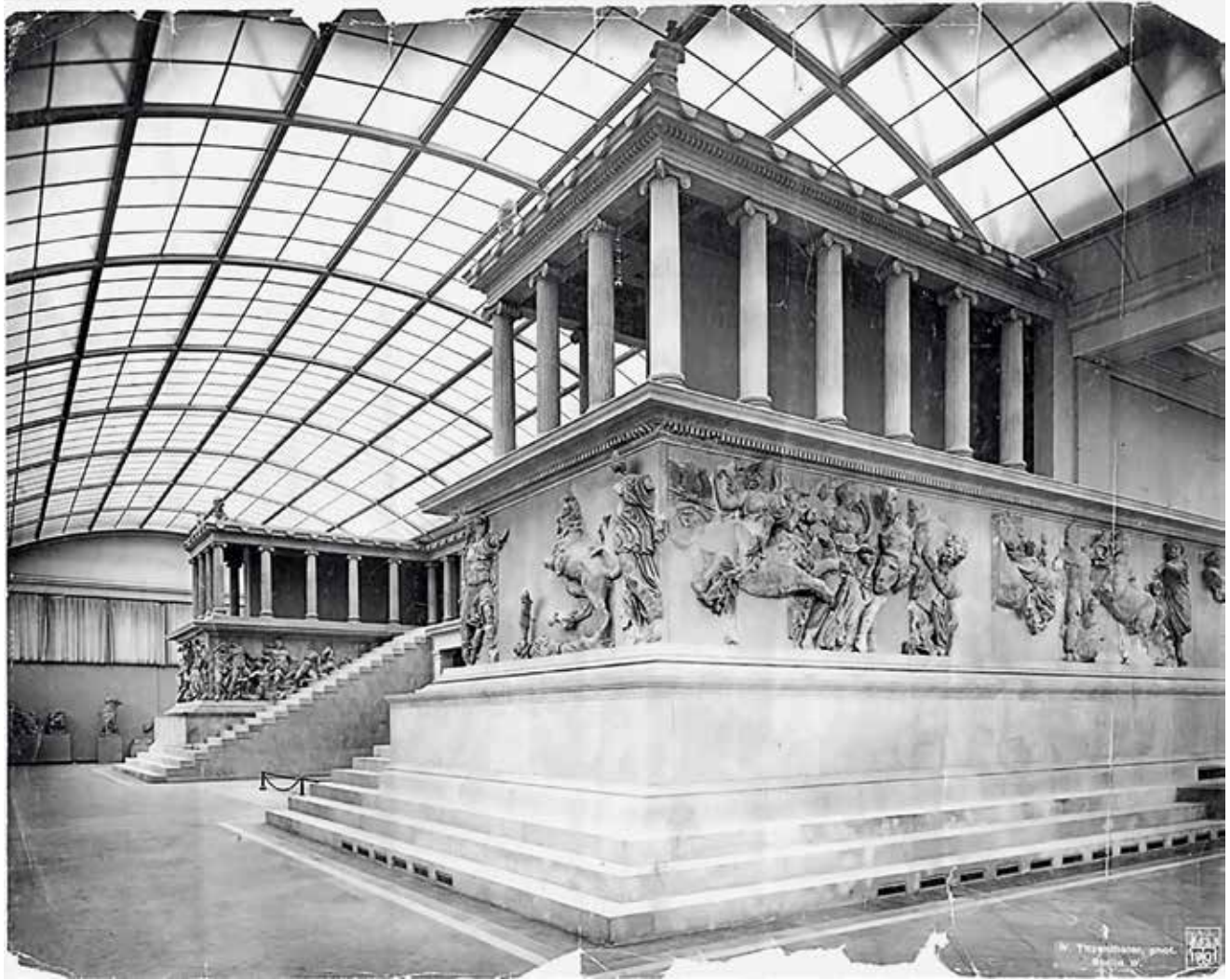
FIG. 2. Old Pergamon Museum (1901–8), Pergamon Altar, view of the reconstructed west facade. Antikensammlung, Staatliche Museen zu Berlin
