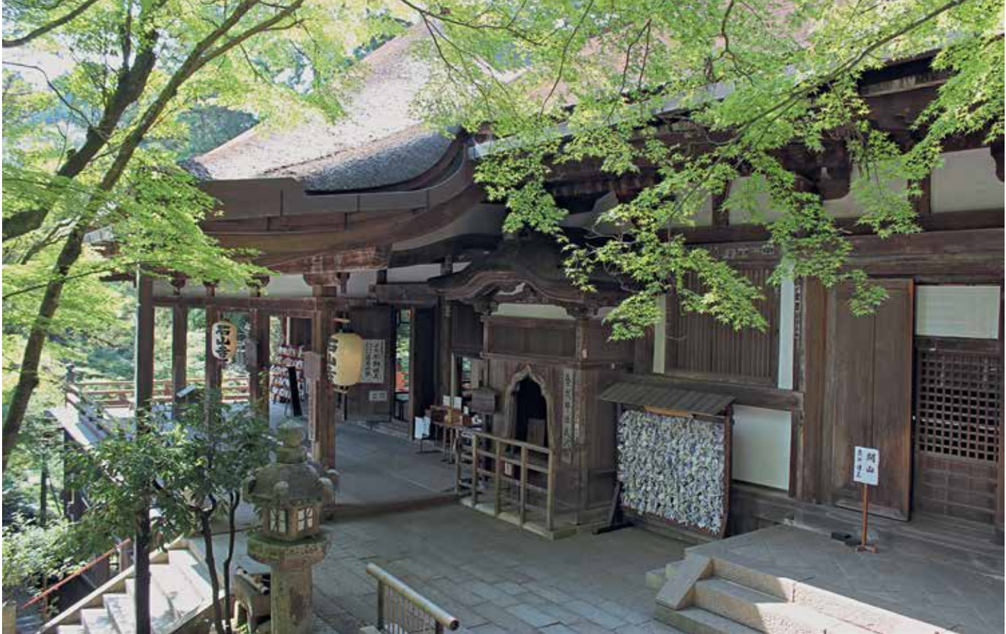
Fig. 54. View of the Main Hall of Ishiyamadera Temple showing the pointed-arch window ( katōmado ) of the Genji Room
