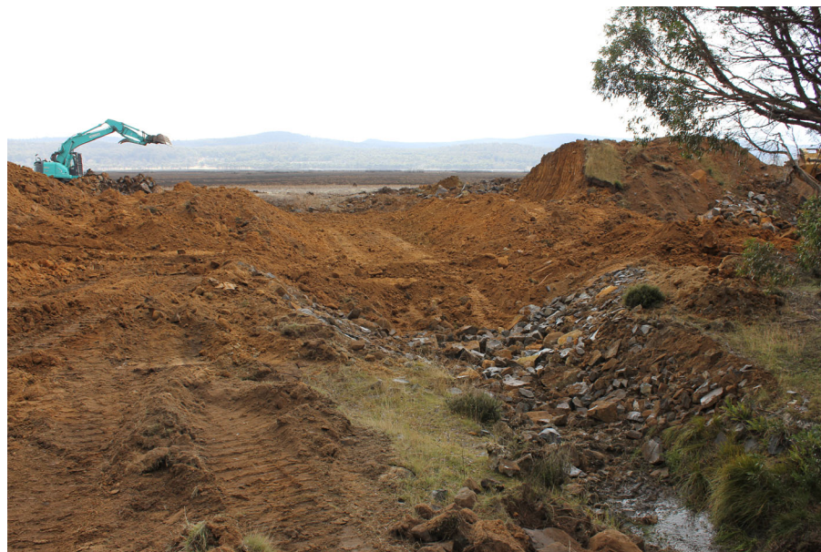
Figure 4. Decommissioning the dam at Lagoon of Islands.
