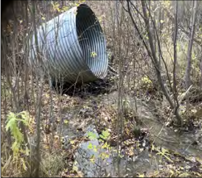
Photo 1. Facing right downstream bank towards inlet
