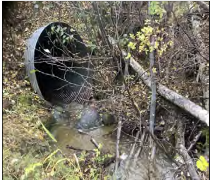
Photo 4. Facing downstream towards culvert inlet
