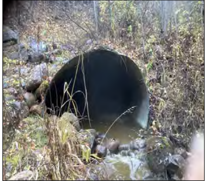
Photo 2. Facing outlet of culvert
