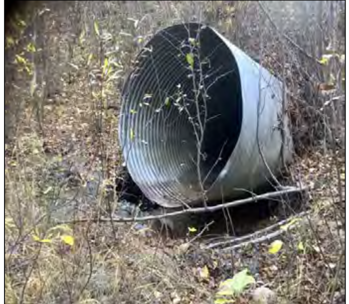
Photo 2. Facing left downstream bank towards inlet
