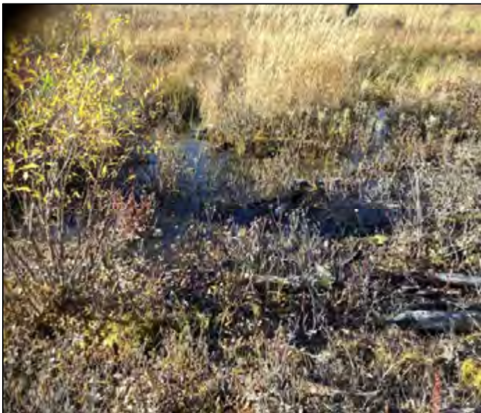
Photo 3. Standing water on west side of existing winter road
