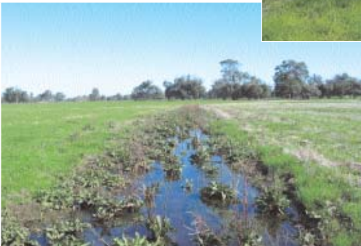
D3 grade foreshore. This drain is approximately 1 metre wide, with very low flows. Due to the low flows, the grasses and clovers are able to hold the bank together and there is little erosion occurring,
