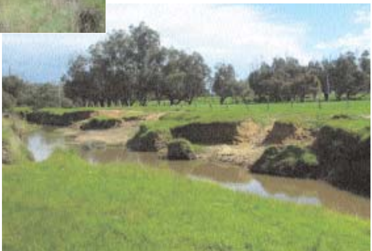
D2 Grade foreshore. No fringing vegetation remains and banks are freely eroding, resulting in massive sediment transport downstream, loss of productive land and serious downstream water quality issues.
