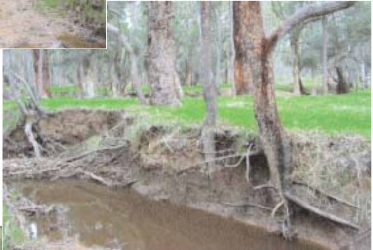
C3 Grade foreshore. Tree roots are barely holding bank in place, with undercutting and subsidence apparent. Only mature trees remain, with no regeneration of local species, as a result of stock access and weeds. These trees are all doomed to be undermined eventually unless supported by revegetation projects using a variety of local species.
