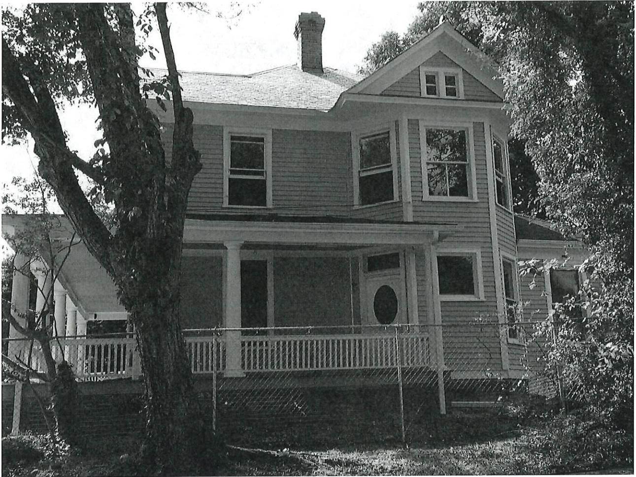
Figure 2: Right side elevation of William A Curtis House ( Other Name: Villa Florenza). 1415 Poole Rd, Raleigh, NC 27610. Photo by Xin Rui Xia in July 2017.
