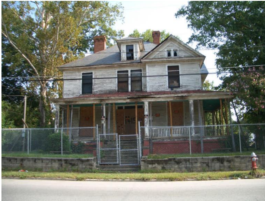
Overall front view
