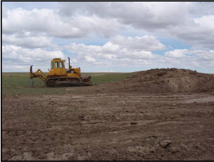
Bulldozer filling-in a pit in a playa to restore natural hydrology
