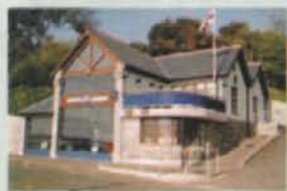
Above – Penarth's new lifeboat station before, during and after construction.
