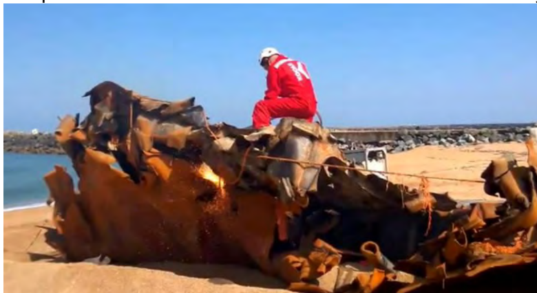
Torch cutting © Bertrand Lapegue
