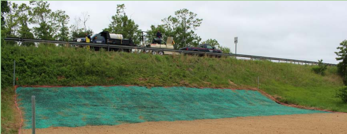
Figure 3.6 Hydroseeded slope along US Route 6.
