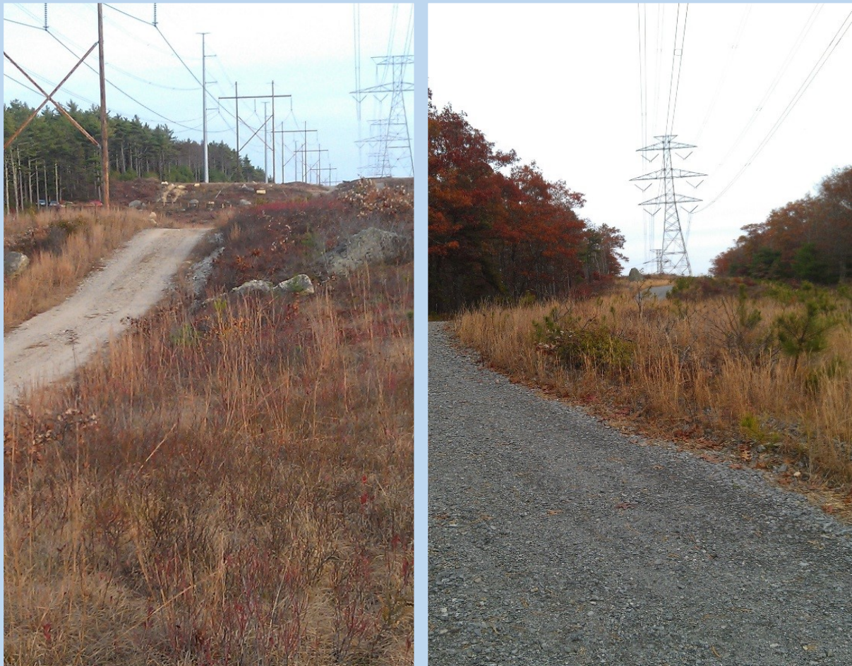
Figure 1.2 Railroad and power-line rights-of-way corridors with poor, dry soils, regular vegetation management, and full sun exposure—similar to the harsh environments along roadsides – demonstrate the natural recovery from disturbances and formation of sustainable grass communities. Photos of power line right-of-way in Myles Standish State Forest, Plymouth/Carver, Massachusetts, with established native grassland vegetation.
