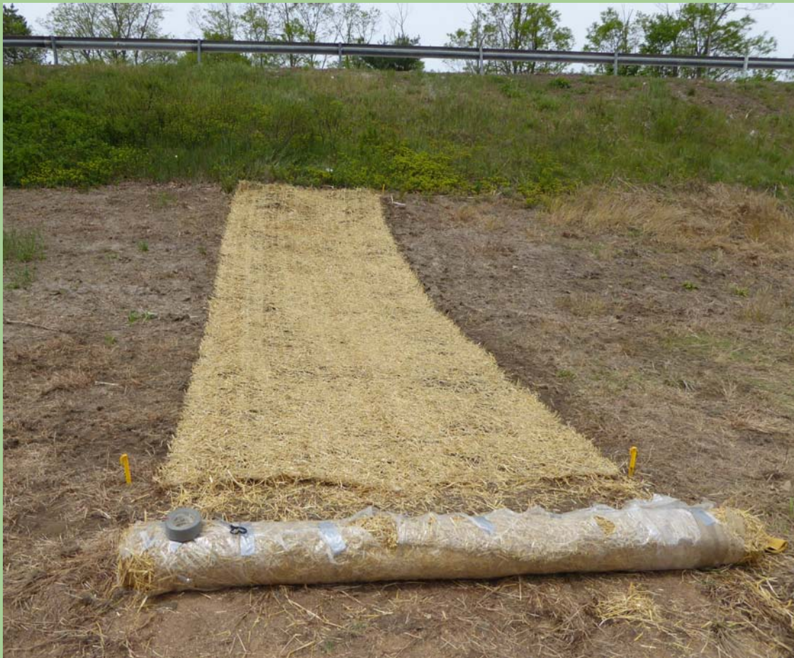
Straw netting erosion control blanket on slope along US Route 6.
