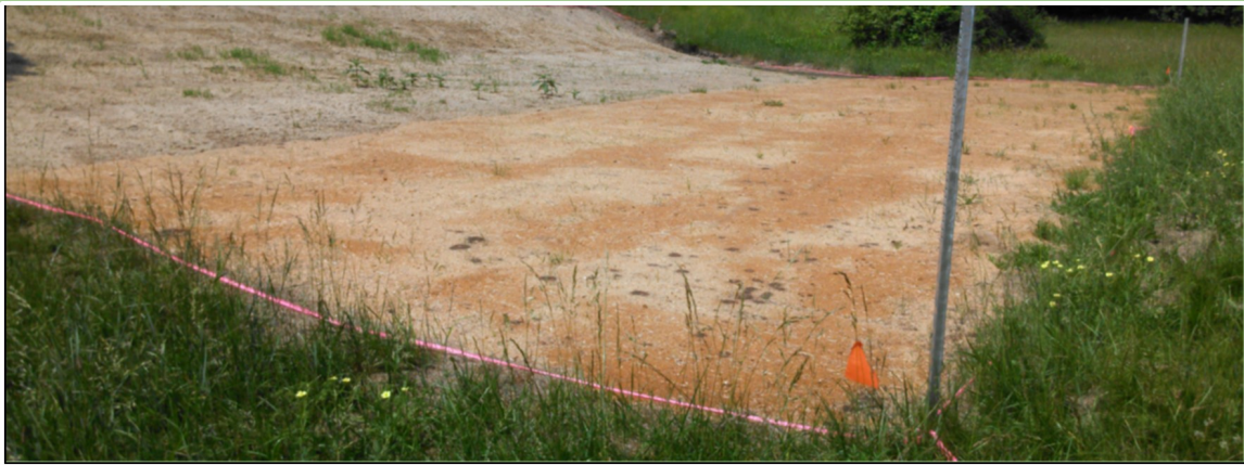
Figure 3.8 Sawdust mulch mixed with native seed and spread evenly along ground.
