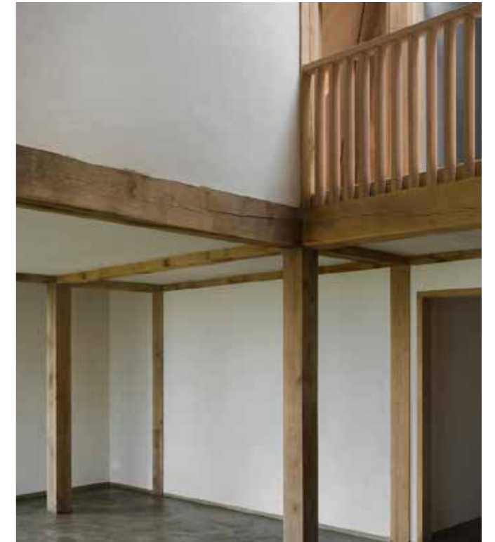
'Kalkhennephuis' by Werstatt (Holland): Hempcrete infill with lime finish
