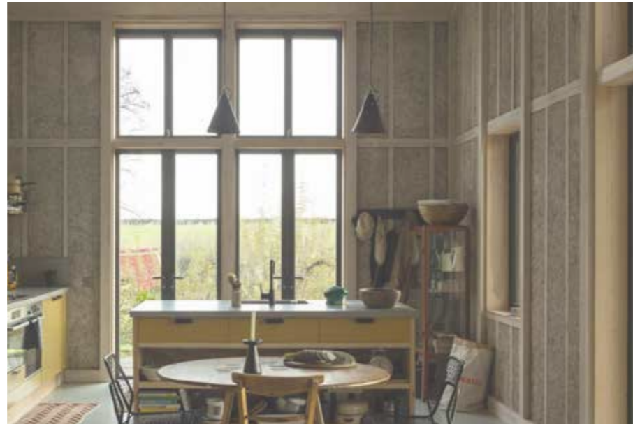
Flat House' by Practice Architecture (London): Hempcrete infill exposed to the interior
