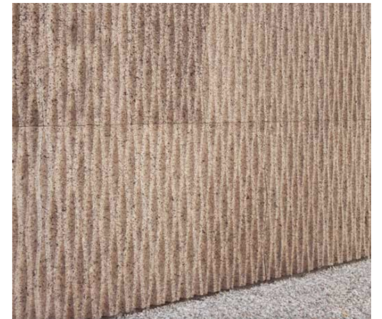
'The House of Wood, Straw and Cork' by LCA Architetti: CNC milled cork facade
