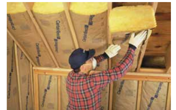
Installing fibreglass insulation
