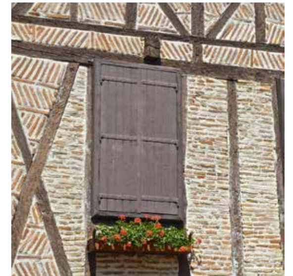
Timber frame with brick infill
