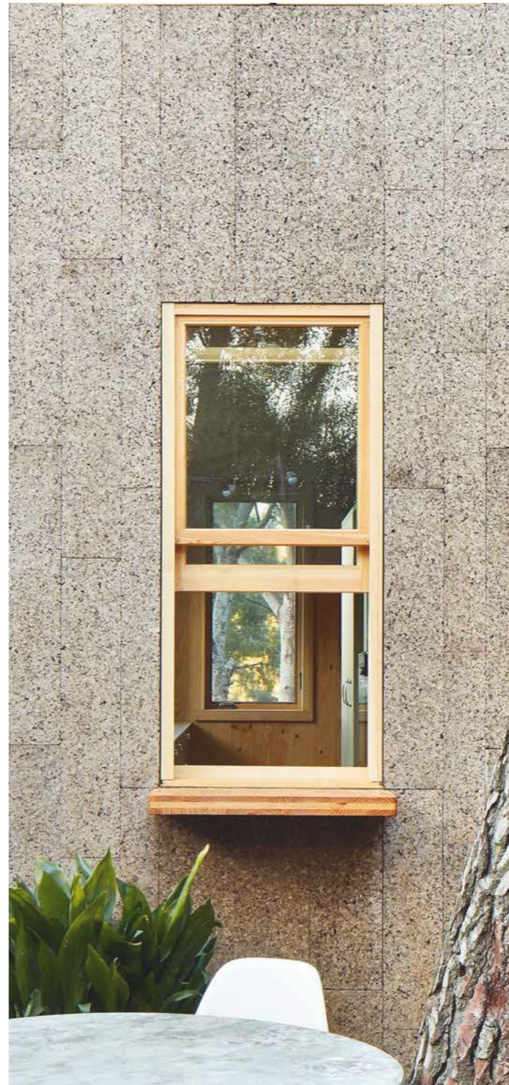
'Two Cork Houses' by López Rivera Arquitectos: Cork cladding
