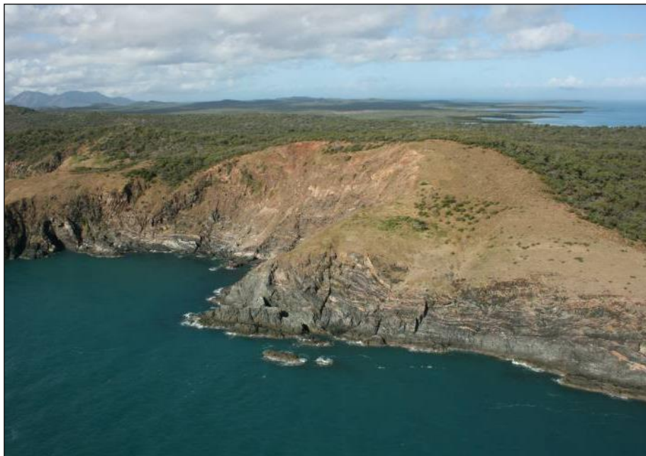
Figure 2-4 Rocky shores along Townshend island (© Copyright, DoD)
