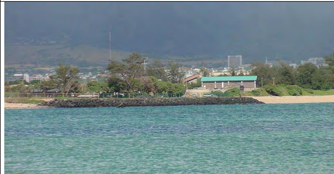
37d. Wastewater Treatment Facility Revetment
