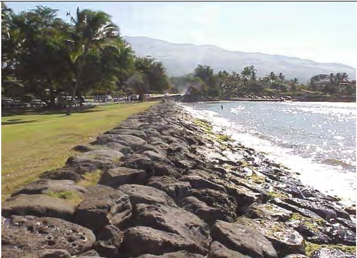
39d. Kalama Park Revetment
