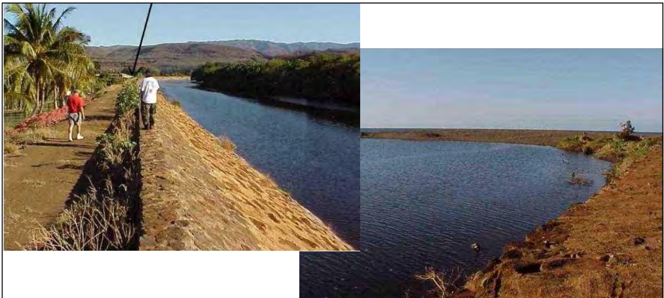
Figure 8. Waimea River Flood Control Project Photos
