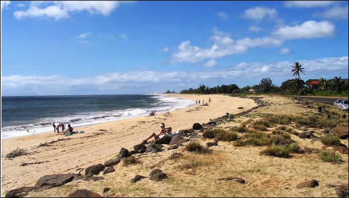
33a. Kekaha Beach Revetment
