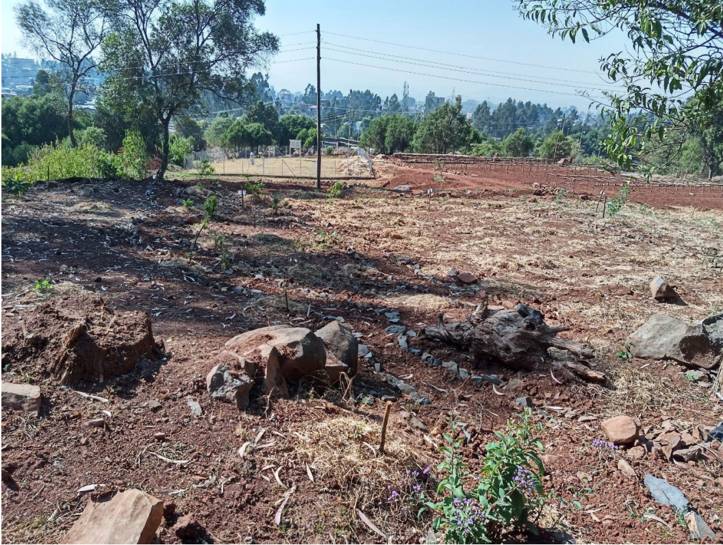
Fig. 7. Site clearance and preparation done for Red List Theme (Oct. 2020)
