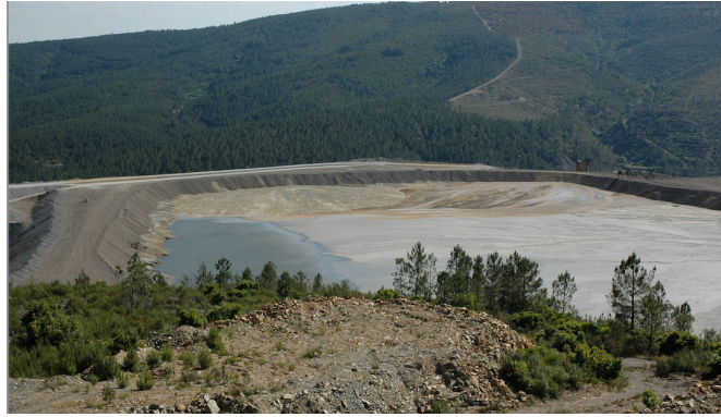
Figure 2. Rejected fraction of the sludge circuit at the Panasqueira mine (Covilhã, Portugal).
