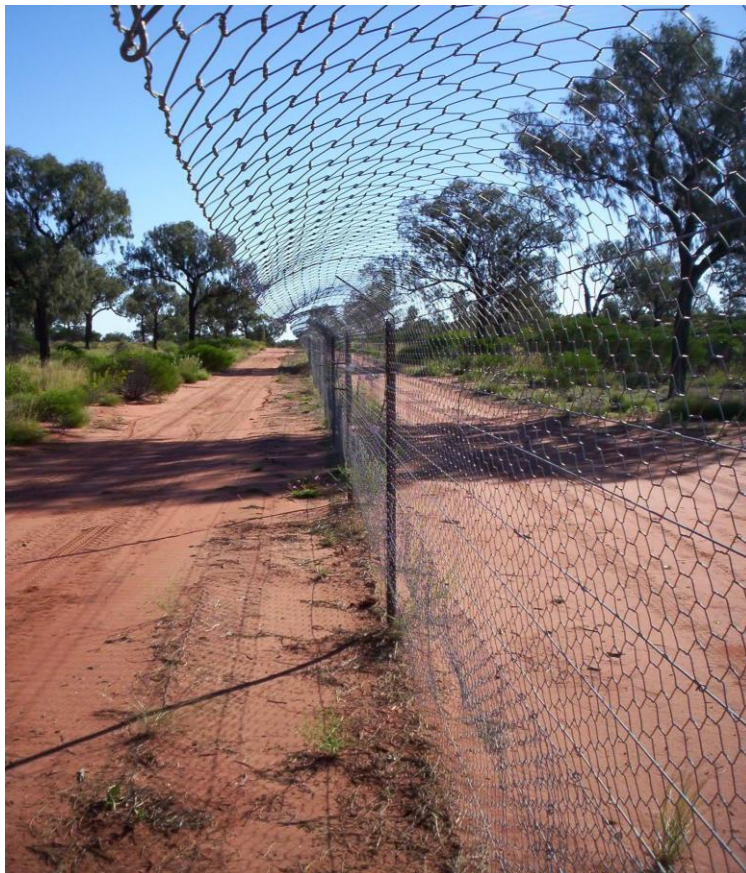
Figure 1.11 The UKTNP mala enclosure predator-proof fence
