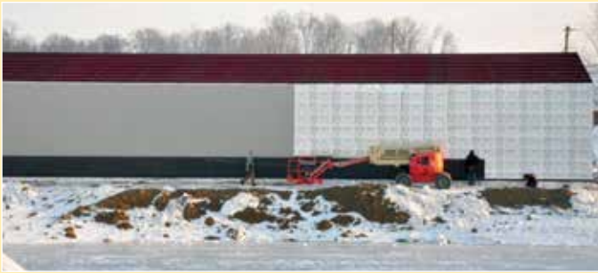
1" WRE 3H+ on walls and roof. PHOTO COURTESY OF TBC
