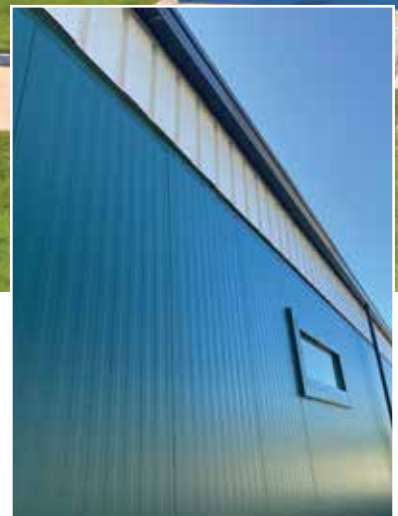
The prior golf barn had canvas walls, which have now been replaced by IMPs. PHOTOS COURTESY OF METL-SPAN (MBCI)
