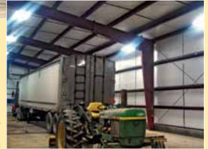
1" WRE 3H+ on finished walls and ceiling. PHOTO COURTESY OF TBC
