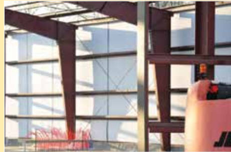
1/2" RRE 3H+ placed under concrete radiant heat floor. PHOTO COURTESY OF TBC
