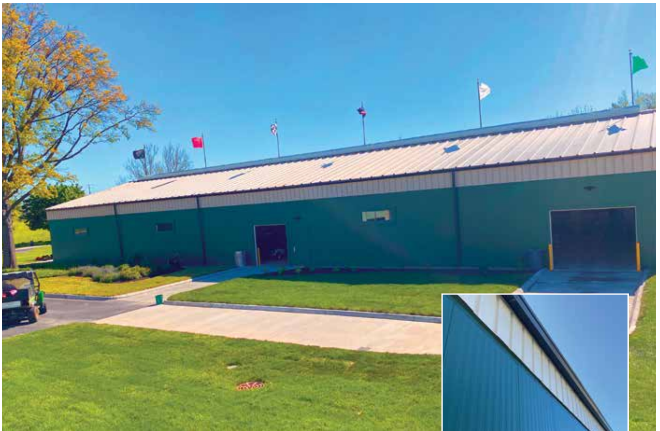
The prior golf barn had canvas walls, which have now been replaced by IMPs. PHOTOS COURTESY OF METL-SPAN (MBCI)
