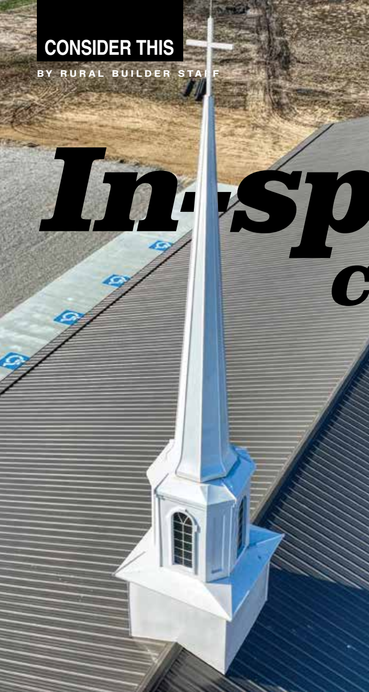
Victory Community Church Spire, Washington, Indiana. PHOTOS COURTESY OF GRABER POST BUILDINGS
