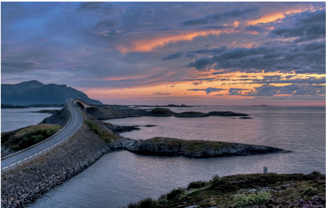
Fig. 125: Storseisund Bridge, part of the Atlanterhavsveien .
