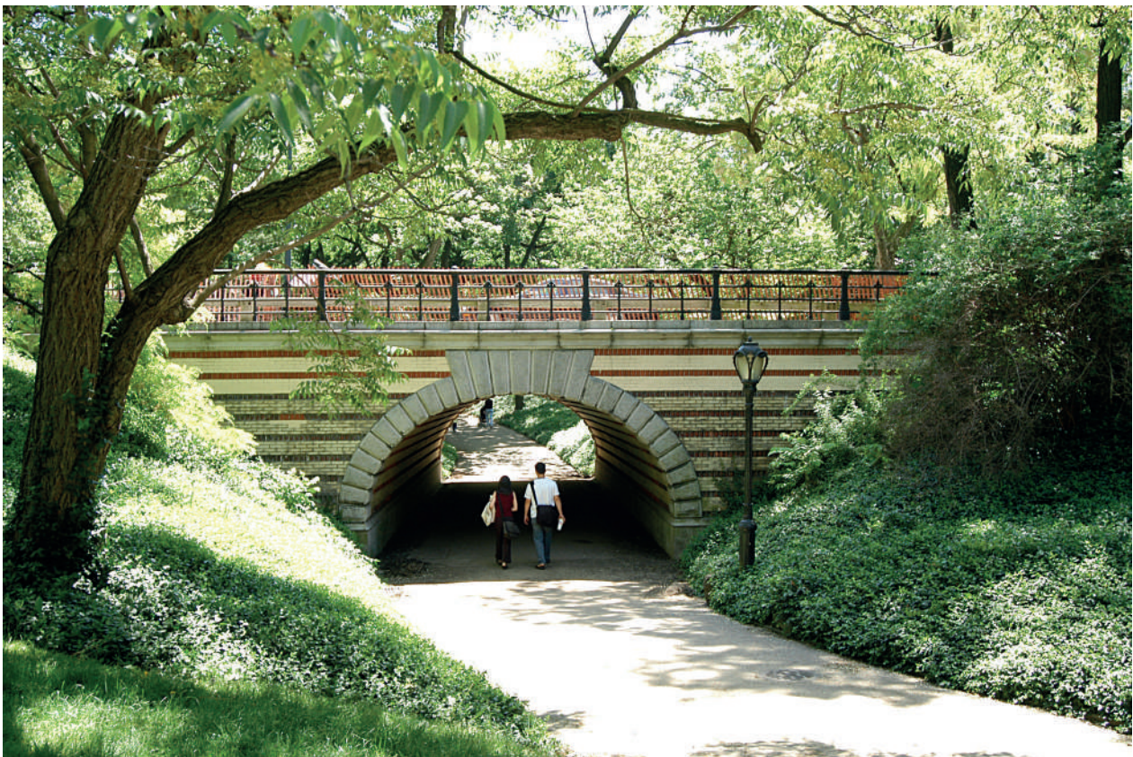
Fig. 87: Separate ways for carriages and pedestrians in Central Park. Bridge designed by Calvert Vaux.
