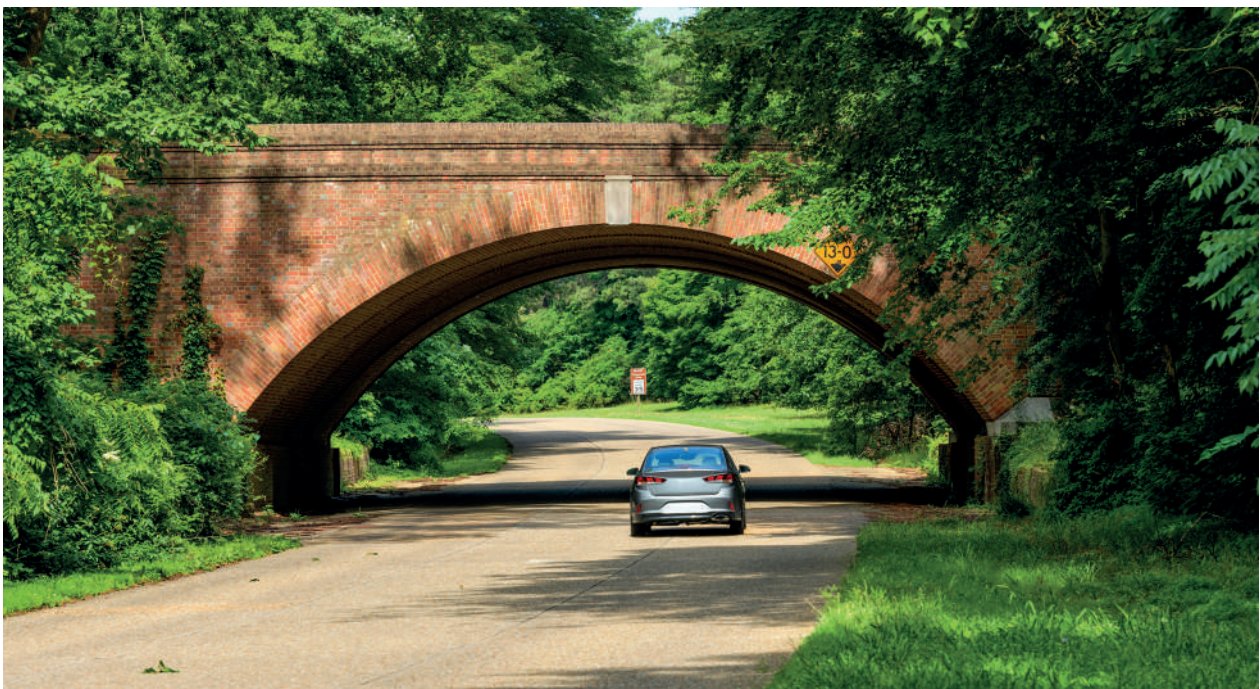
Fig. 90: Brick underpass on the Colonial Highway.
