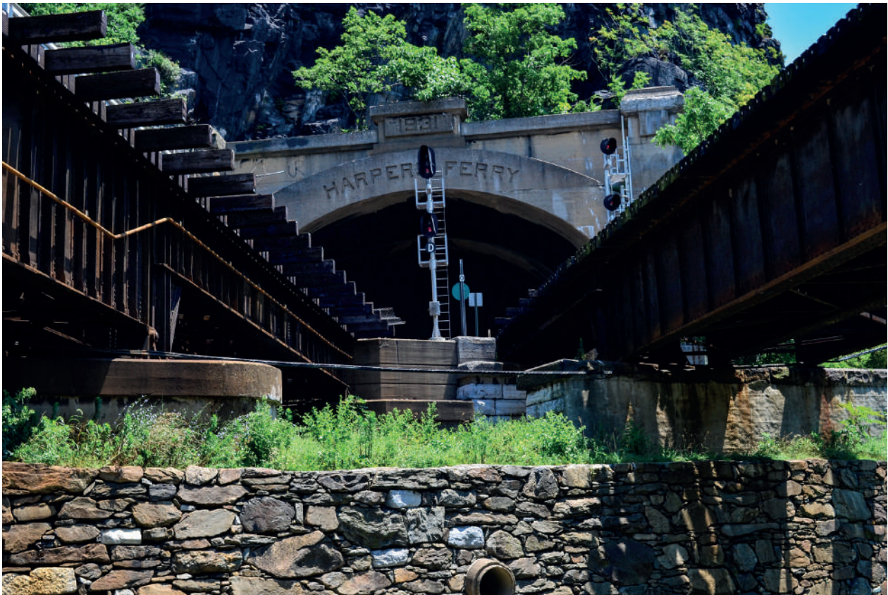
Fig. 36: B&O Railroad Bridge in Harpers Ferry, West Virginia.
