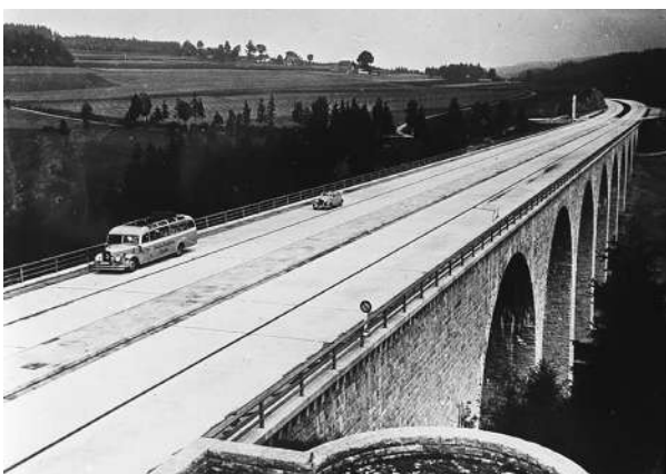
Fig. 66: Bridge over the river Saale at Hirschberg, 1938-1940.
