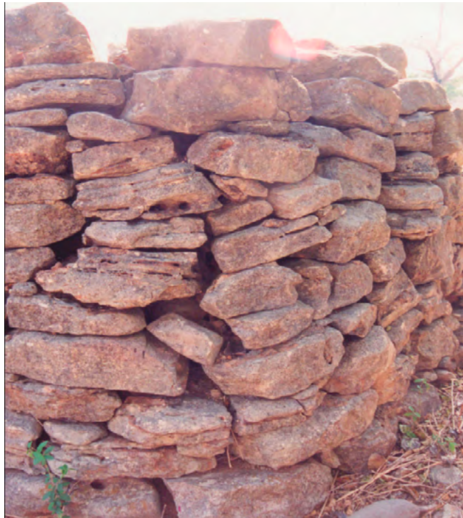
Fig. 8. Face of buttress at Manyikeni stone enclosure. The low quality construction can be observed due to the use of limestone compared with granite.
