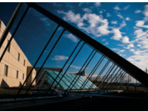
Second annual employee sustainability photo contest winner submitted by Shelli L. Driscoll, from Trane, Knoxville, TN. Trane collaborated with FLS Energy to create one of the largest solar thermal systems for domestic hot water in the United States.
