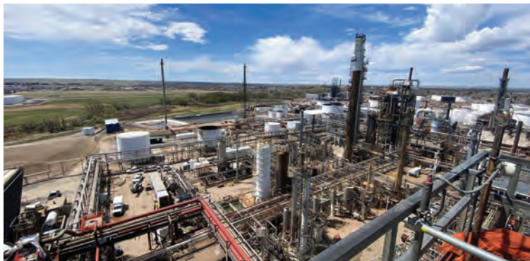
HOLLYFRONTIER CHEYENNE RENEWABLE DIESEL PROJECT CHEYENNE, WY, U.S
