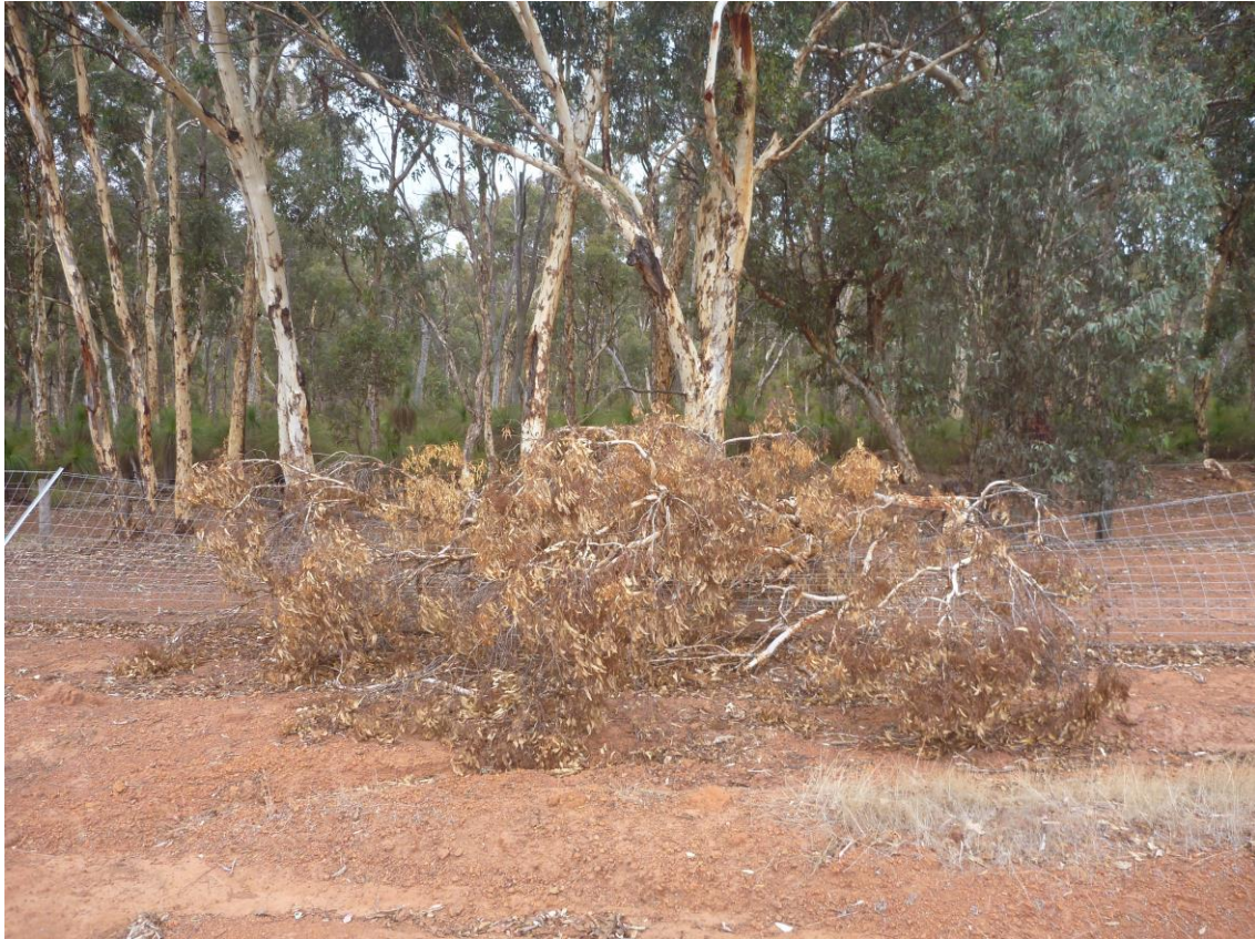
Plate 8: Fence breach reported in the south-eastern corner of the site, April 2019.
