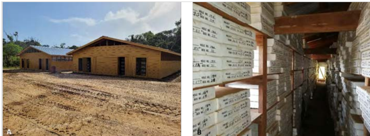
Figure 11-41: Secure core storage (A) and secure wooden core racks (B), inside storage.
