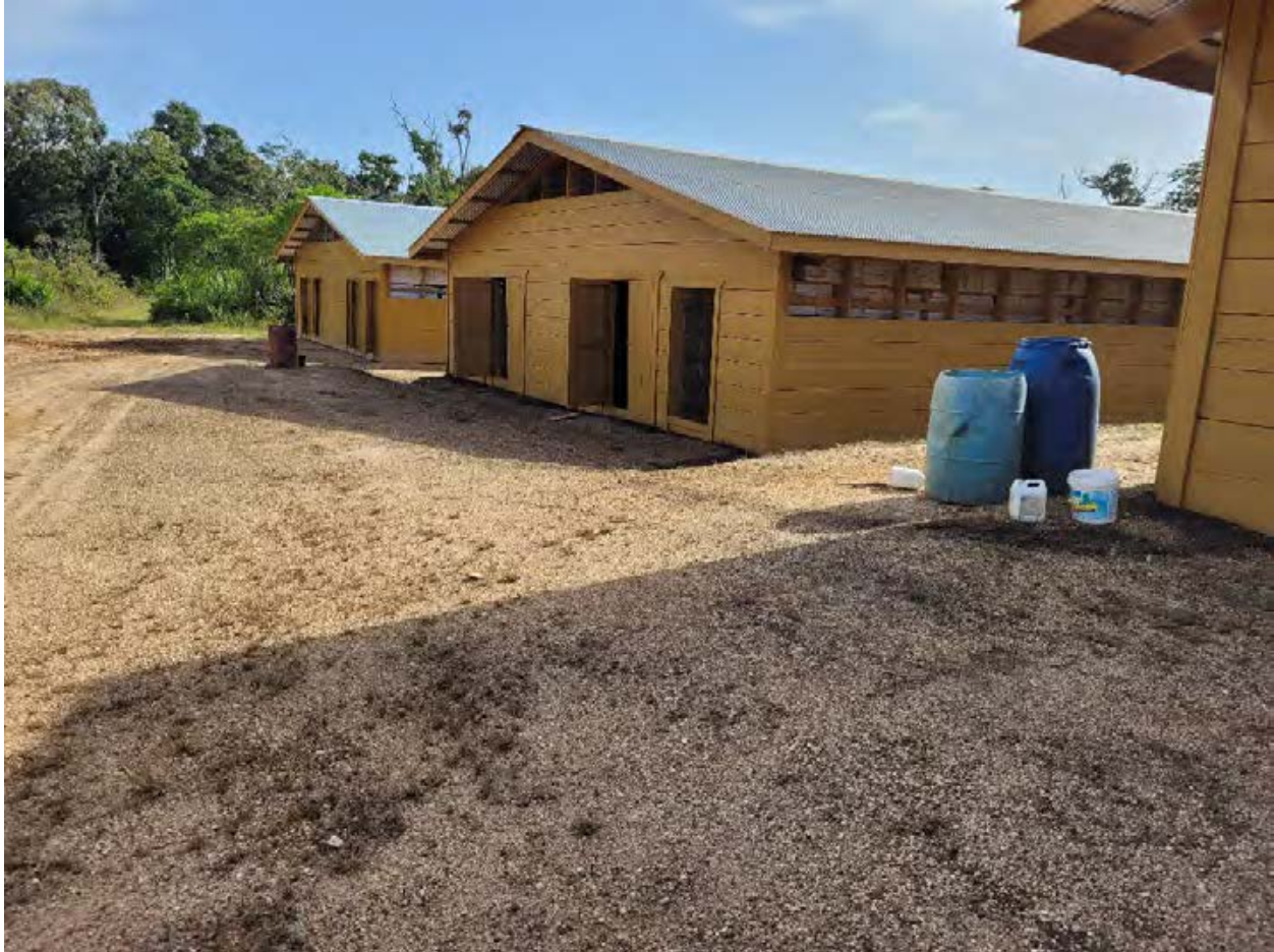
Figure 12-7: Company core storage facility
