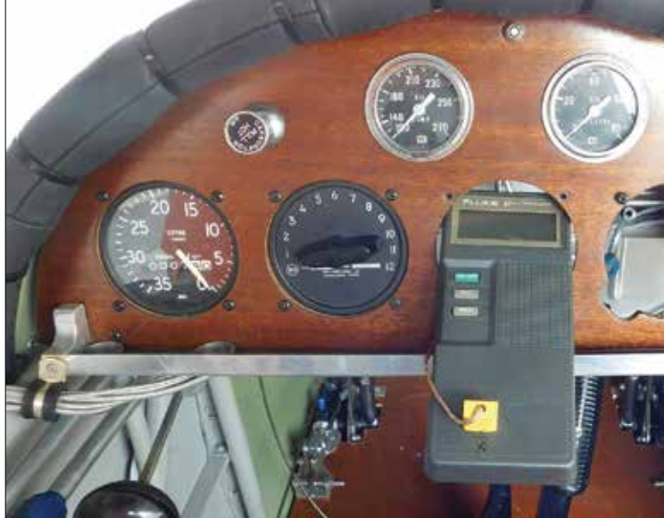
Figure 5: Thermocouple wires come in from the left and the 12-position switch determines which temperature point is indicated on the readout.
