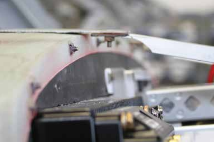
Click Bond nut plates were used everywhere in their Sportsman. Here they serve to hold the instrument panel to the structure.
