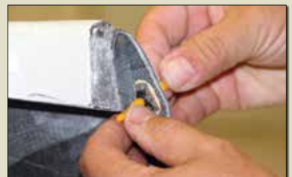
You'll see a nice even bead of adhesive all around the nut plate if you have done it properly. After the adhesive cures, the fixture pops right out.
